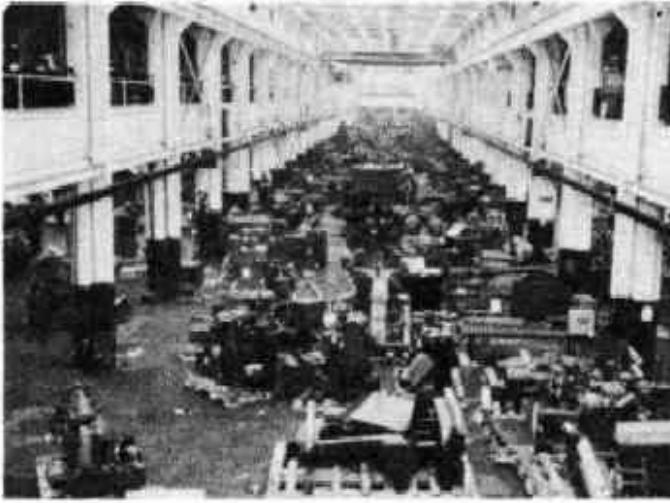
Moving out war production machine tools to make a place for peacetime tools
